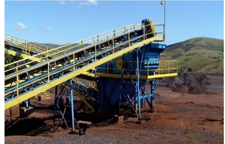
Refurbished existing 1.8Mt per annum plant
