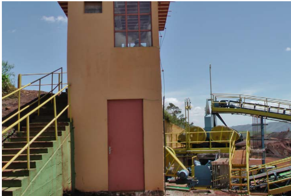
Fig. 2 Operations Control Tower
