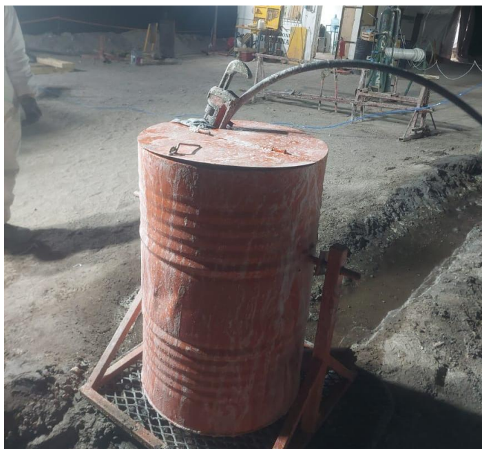
Figure 2 – Brine being recovered from the first DDH-3 packer test into a 200-litre collection barrel.
