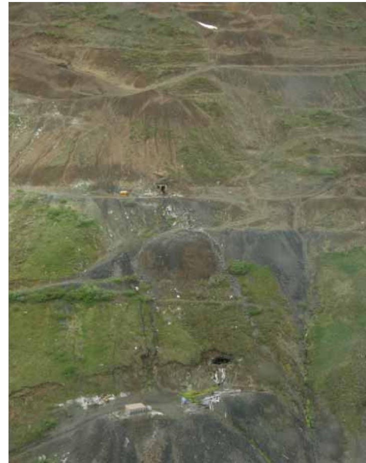
Road access and entries to the historic adit (upper level) and decline (lower level) at the Caribou Dome Copper Project
