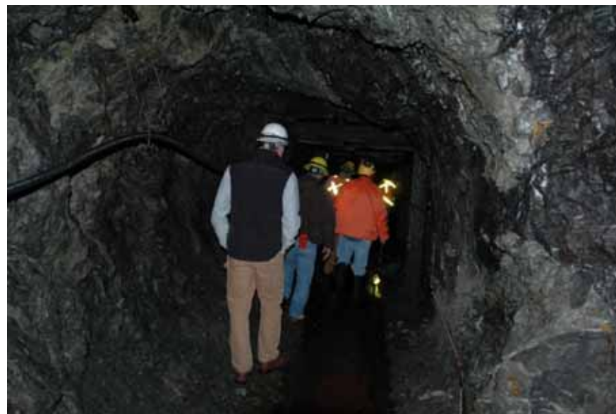
4630 level adit at the Caribou Dome Copper Project. Grey material is an ash unit; black is mineralised sediment
