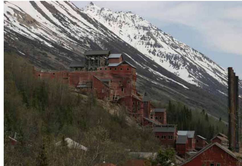
Surface infrastructure at the Kennecott Copper Deposit, Alaska
