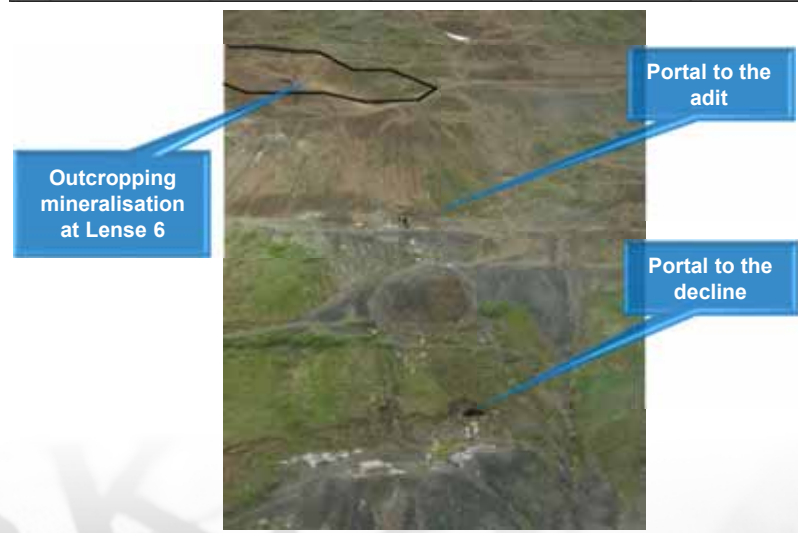
Road access and portals to the historic adit and decline
