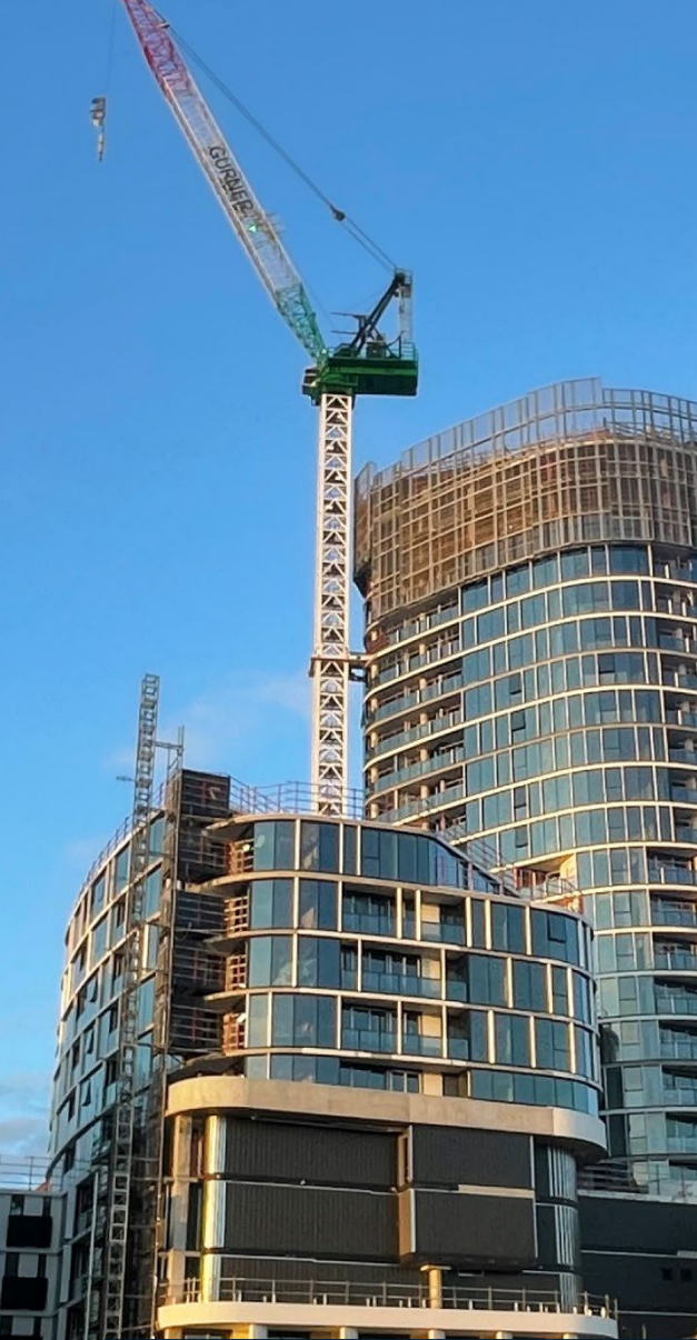
Beach House – 297 units St Kilda, Melbourne To be completed in Q1 2024
