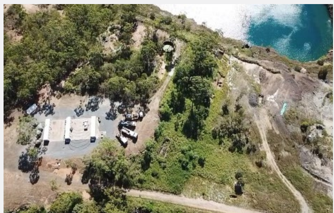
Image 1: Mt Chalmers Site Works Progress, January 2022.
