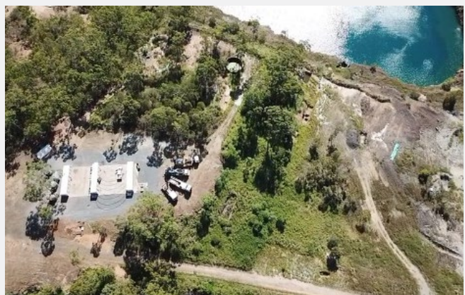
Image 1: Mt Chalmers Site Works Progress, January 2022.
