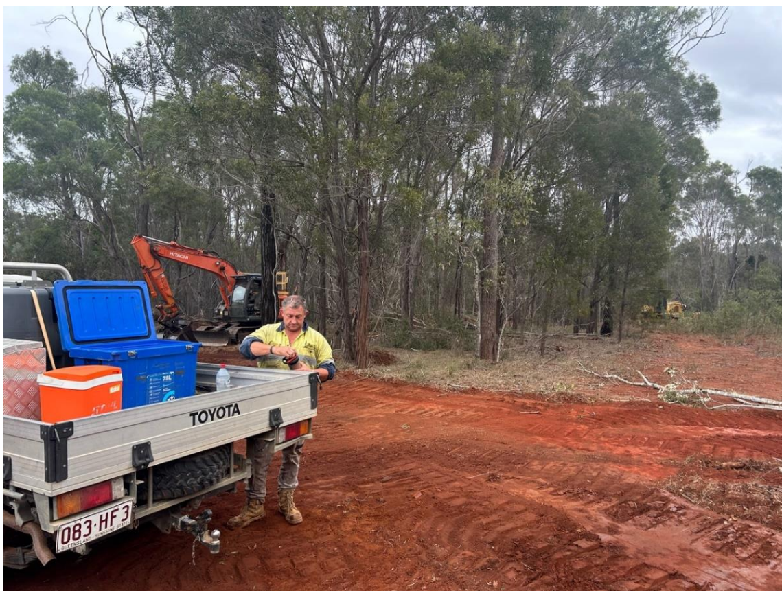
Figure 3: Develin Creek drill pad preparation in progress.
