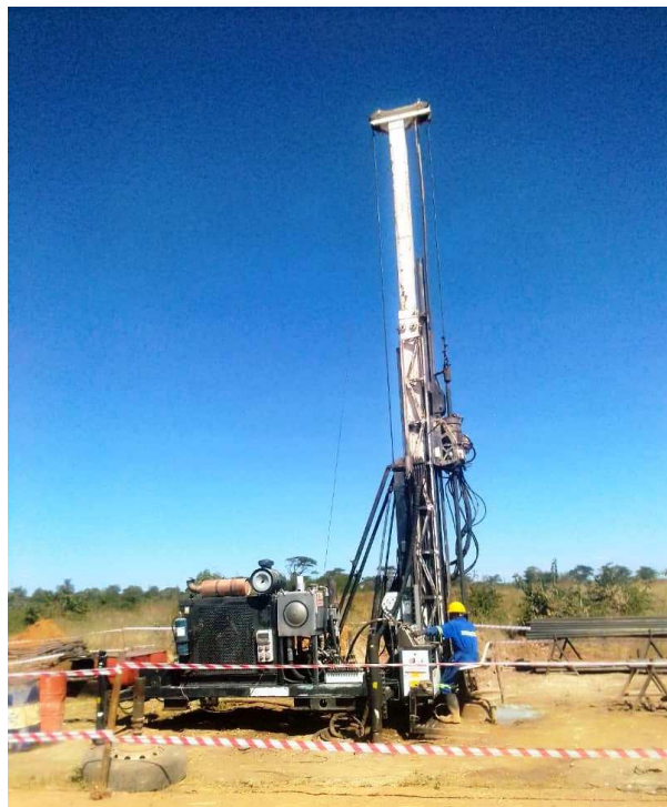
Figure 1. Lonely Mine Gold Project – Diamond Drilling Works
