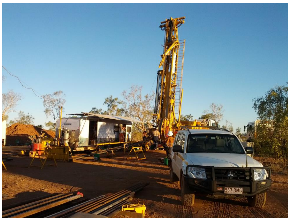
[Figure 1] Maronan Project: Drilling in progress
