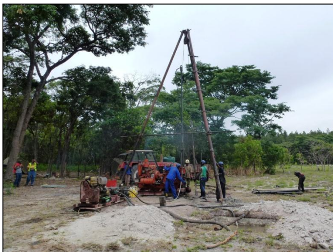
Figure 2. LDD-2 in progress
