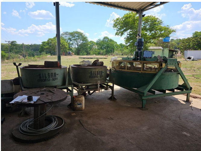
Figure 10: Existing equipment onsite.
