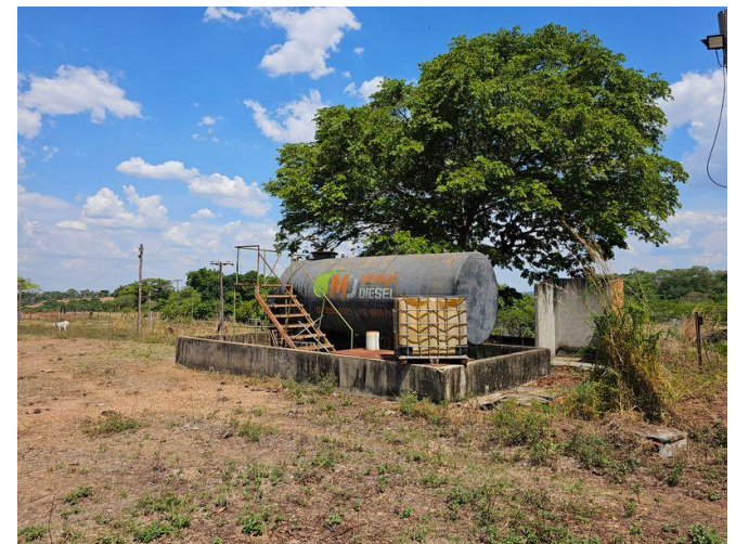
Figure 11: Fuel holding tanks.
