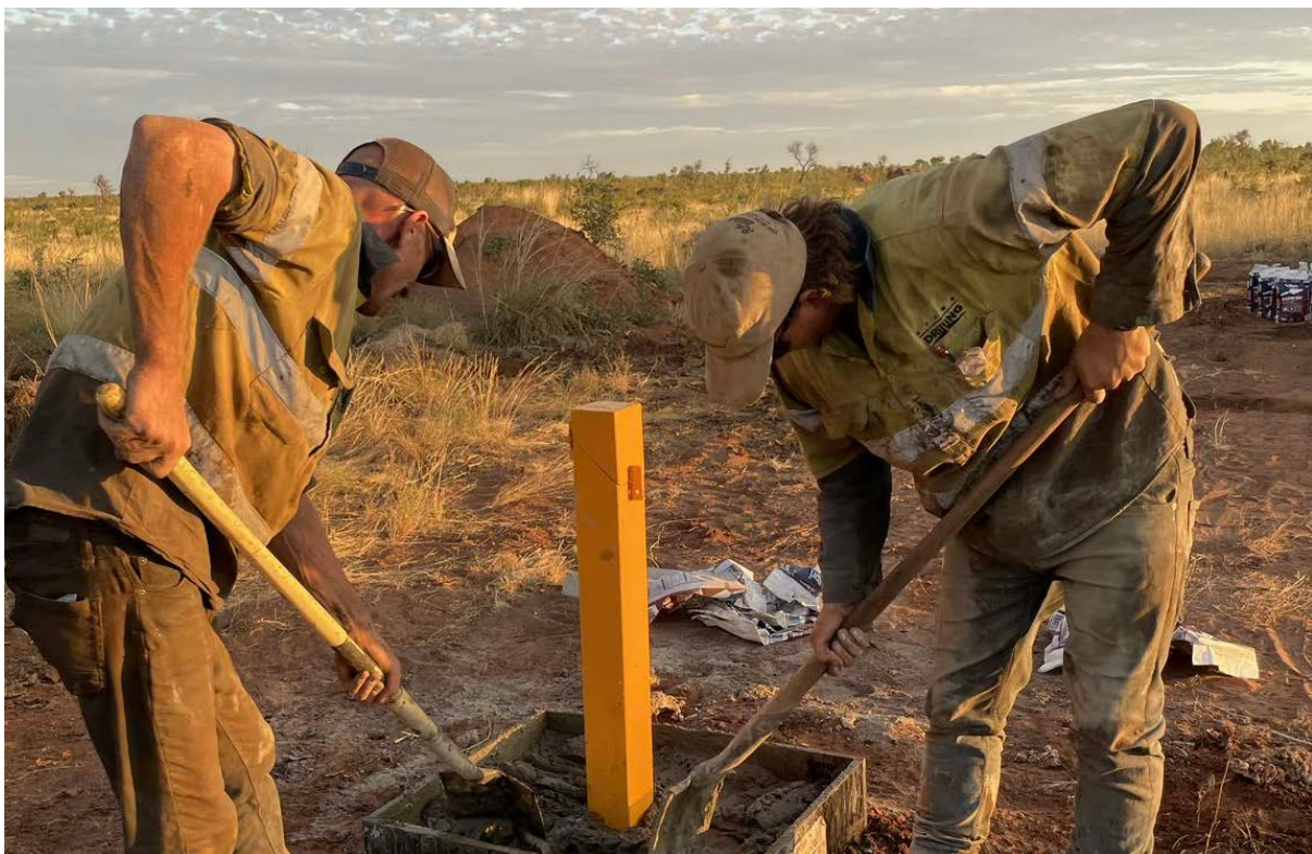
Figure 14-1: Water monitoring bore installation
