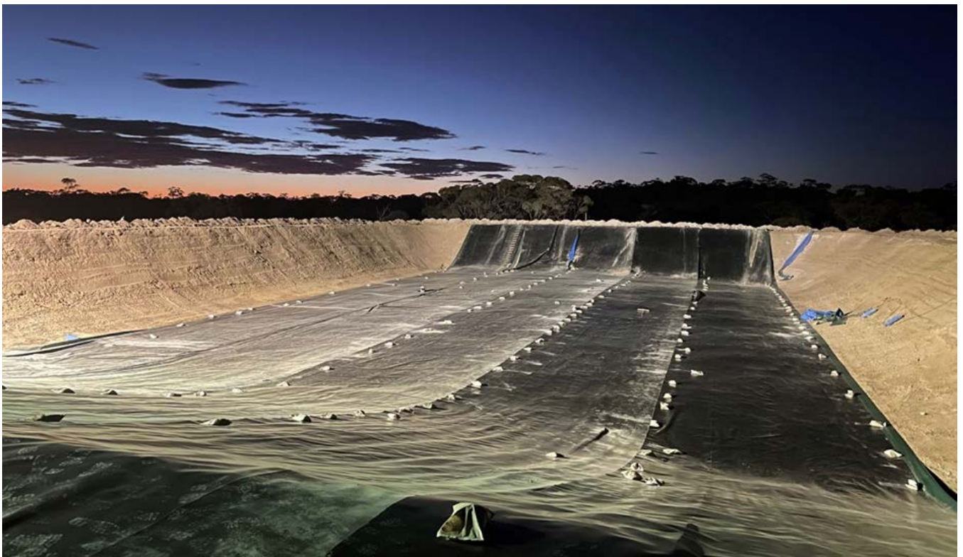
Figure 2: An Eastern Goldfields example of a vat leach pad under construction (source: Vat Leach Consultant)
