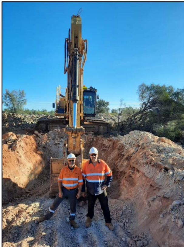
Figure 6: Contractor Lamington Minerals Pty Ltd crew onsite
