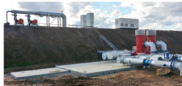
Pump station under construction
