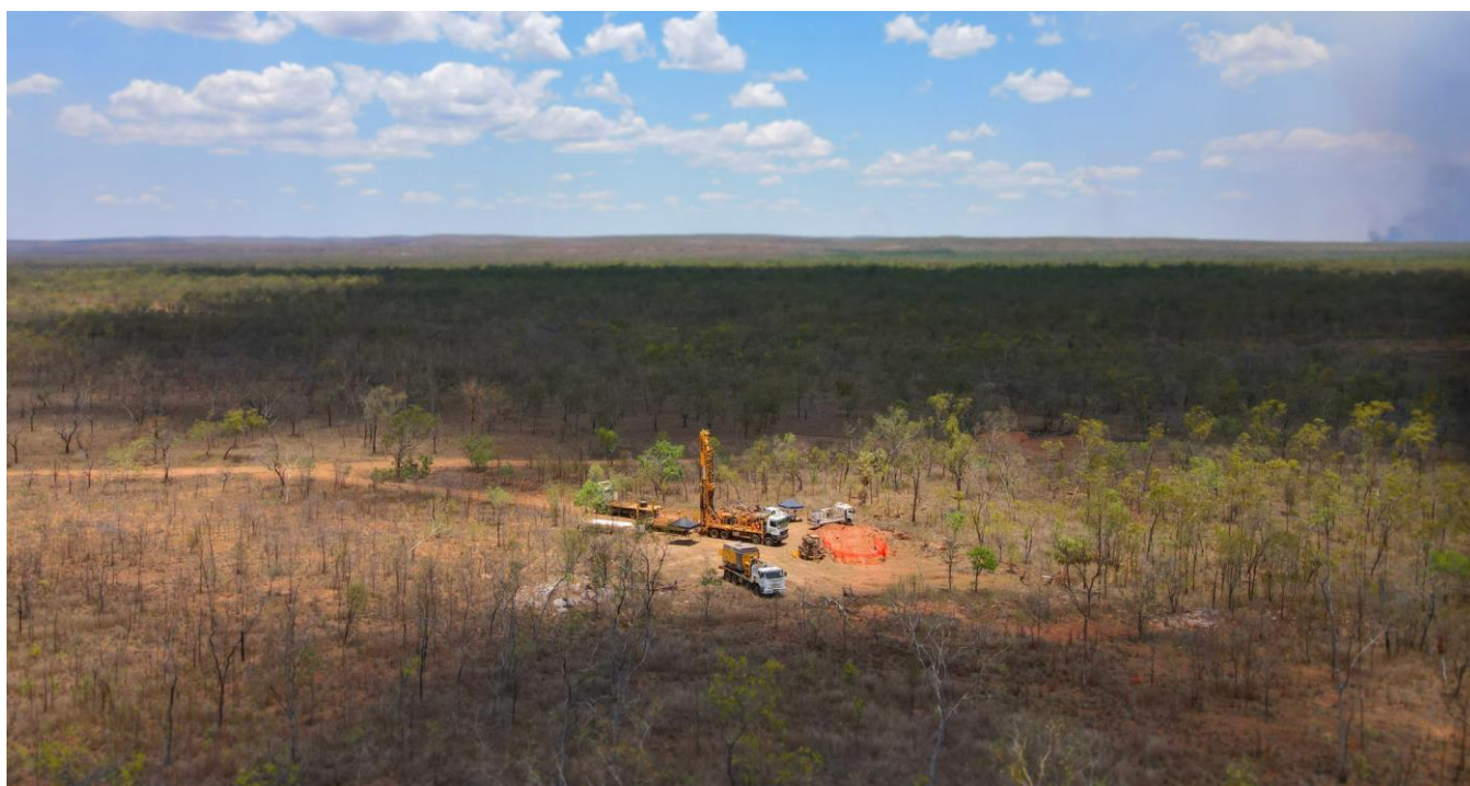
Drill rig set up over the first hole of the 2022 Wollogorang program
