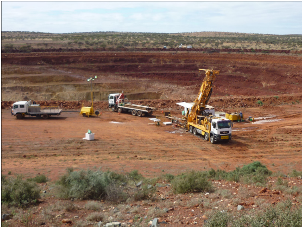
Figure 3. Diamond drilling at Western Queen South March 2012
