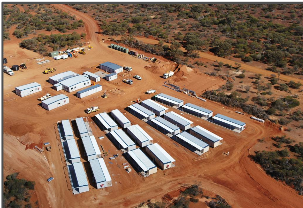
Figure 9: Penny Mine Camp under construction
