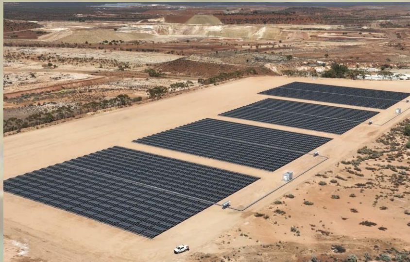
Solar farm at Mt Magnet
