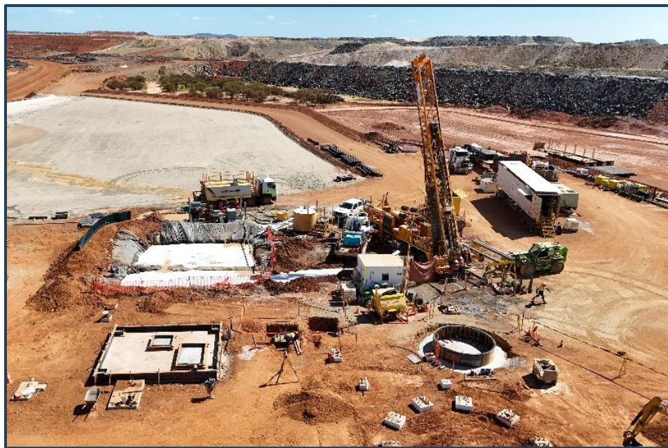
Paste plant construction
