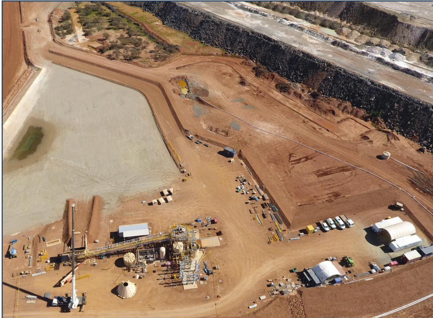
Paste plant construction
