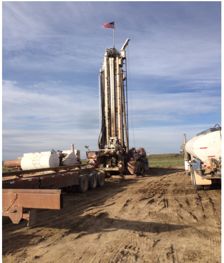
Red Valley: Drilling commences
