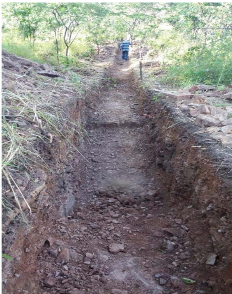
Trenching Work at Mukabe-Kasari
