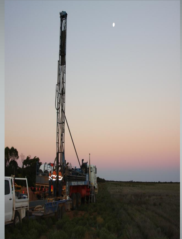
Drilling at Pirie Basin Project
