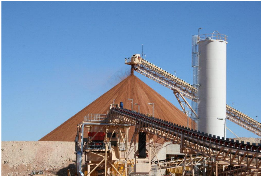
Fine Ore Stockpile
