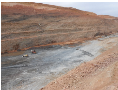
Stage 1-3 looking east (30/6/14) with grade control underway
