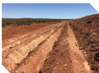
Rosemont NW Waste Rock Landform Rehab-Feb 2016
