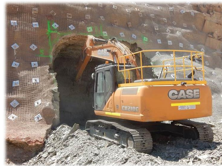
Cutting the Portal
