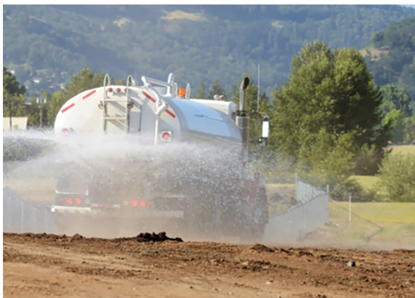
Water cart suppressing dust
