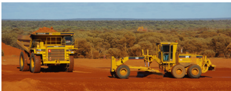
Topsoil conservation during construction – Duketon Operations
