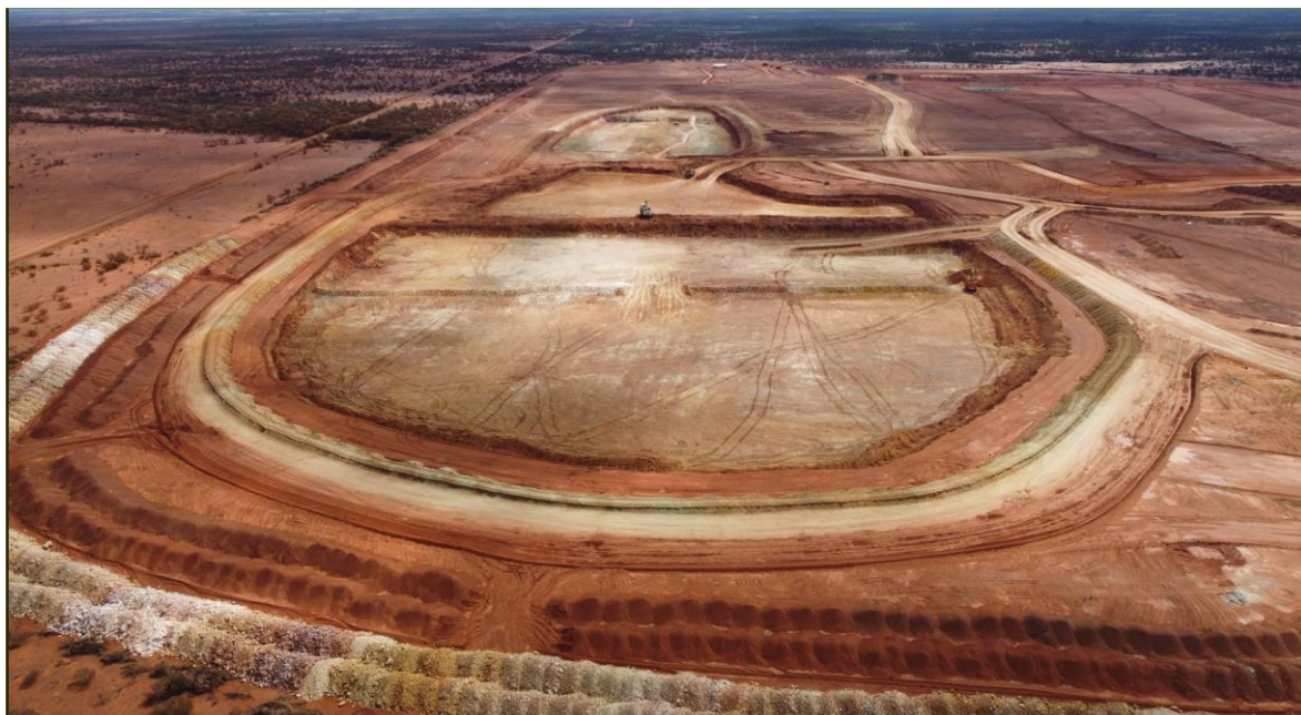
Figure 3: Ben Hur southern pit progress
