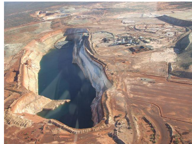
Youanmi Main Pit and Plant
