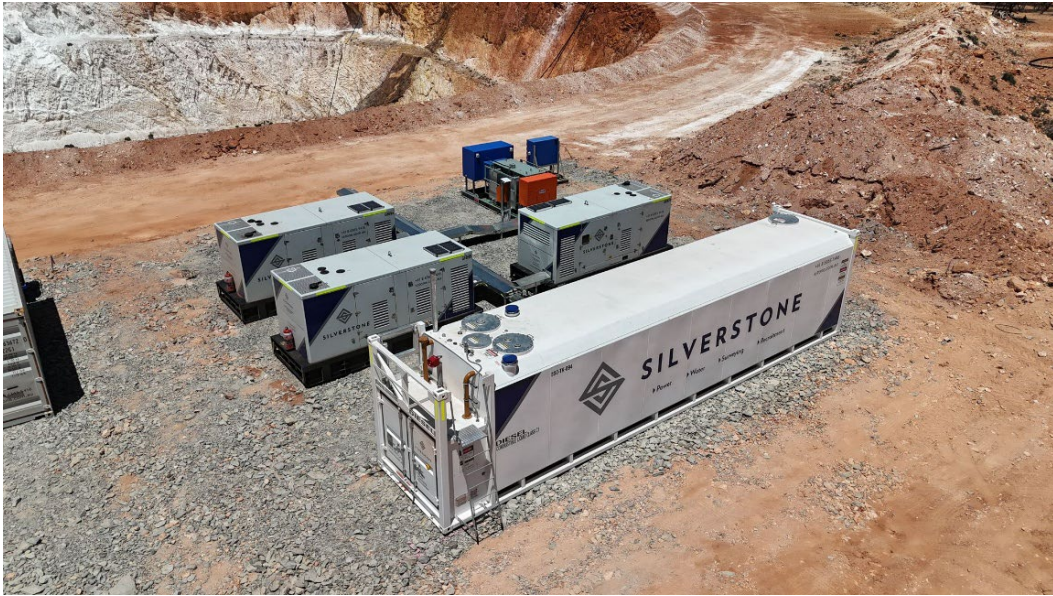
Figure 2 – United North Power Station progressing to commissioning
