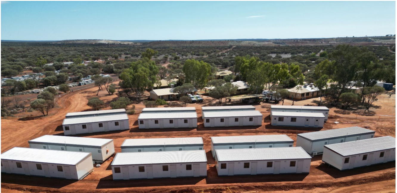
Figure 4 – Phase 1 Camp Expansion works advancing
