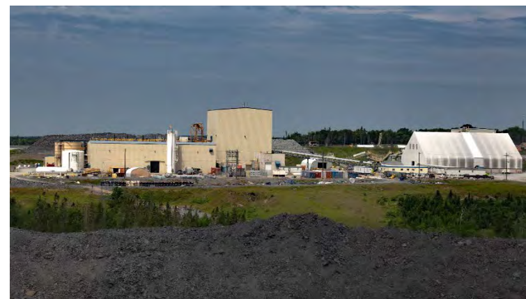
Touquoy processing plant
