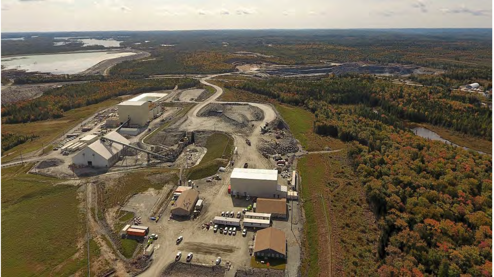
Touquoy processing plant, with open pit and tailings facility in background
