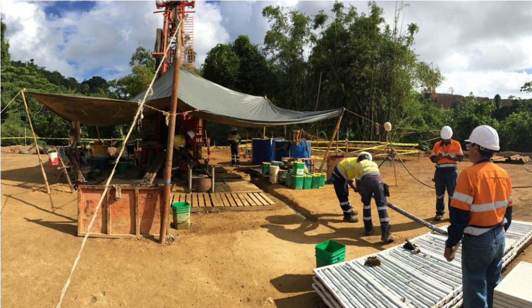
Oxide exploration drill rig at Simberi
