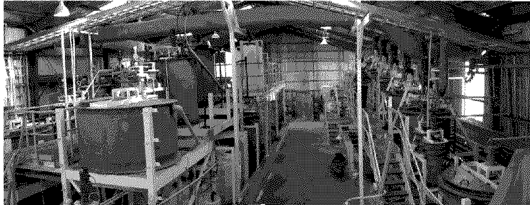
Above: IHM Demonstration Plant under construction during June 2005
