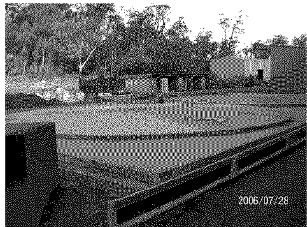
Figure 6: Storage Tanks Area near Intec Hellyer Mill – concrete bases complete
