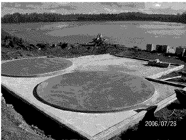
Figure 5: Shore Tanks Area near tailings dam – concrete bases complete
