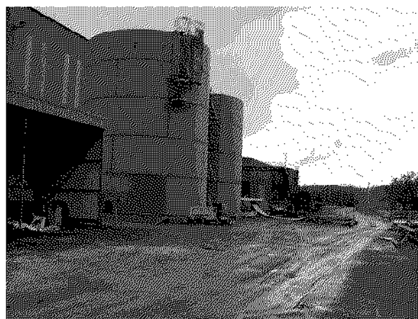
Figure 8: Storage tanks under final assembly adjacent to Intec Hellyer Mill.
