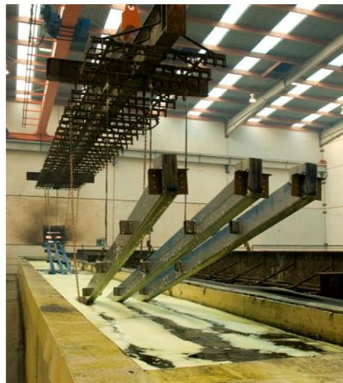
Figure: An acid pickling bath prior to hot-dip zinc galvanising
