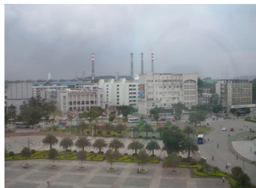
Figure 2: Distant photo of part of Liugang's steelmaking plant taken by Dr Andrew Tong from his room in the hotel owned by Liugang during Intec's recent site visit.
