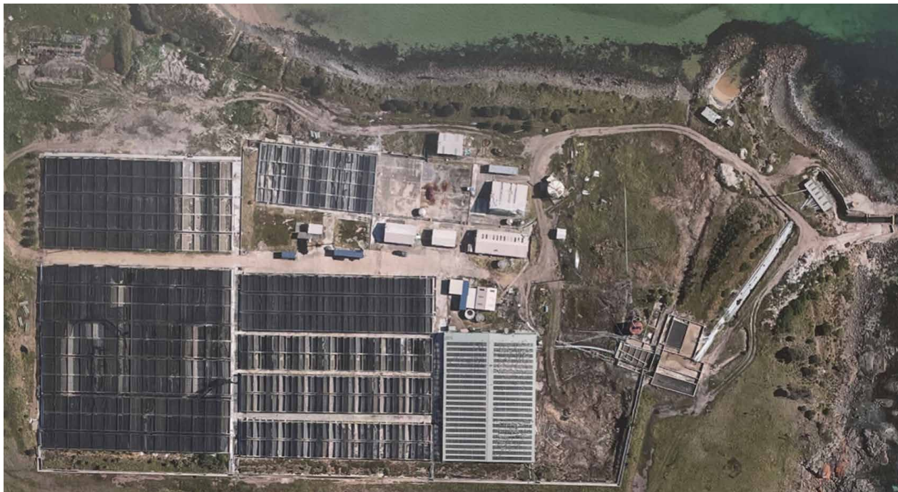
Figure 3.4 – Sea Forest facilities in Swansea, Tasmania
