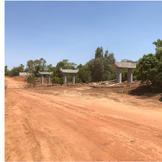
Keep River Bridge Road – Completed Pylons
