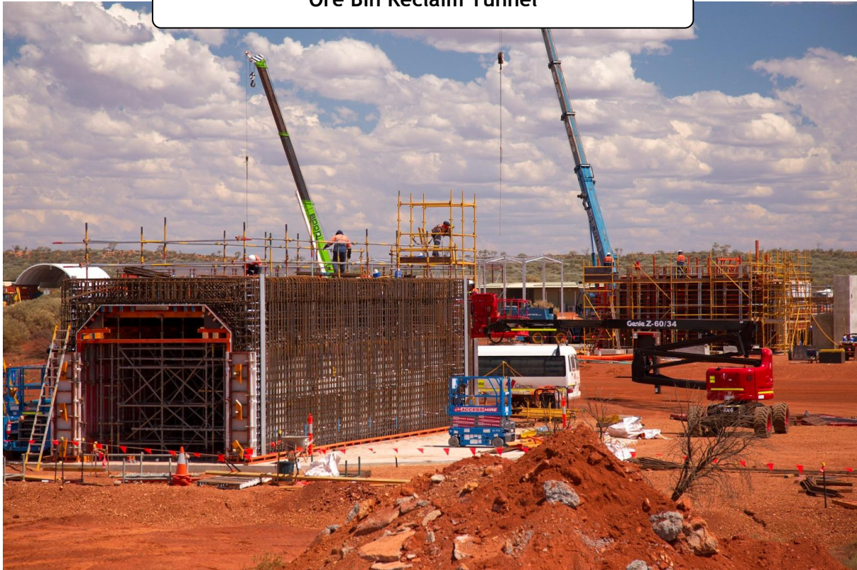
Ore Bin Reclaim Tunnel
