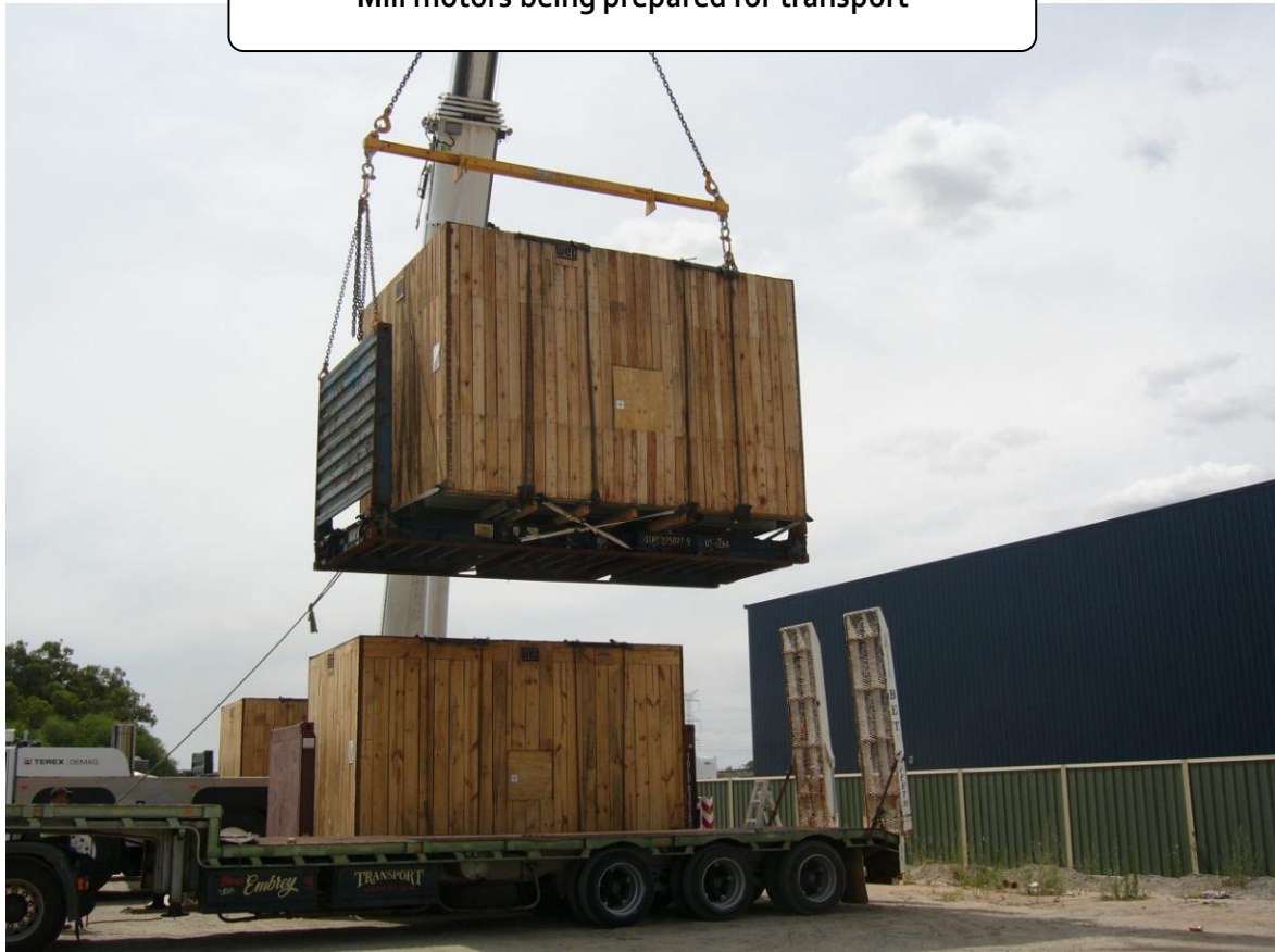
Mill motors being prepared for transport
