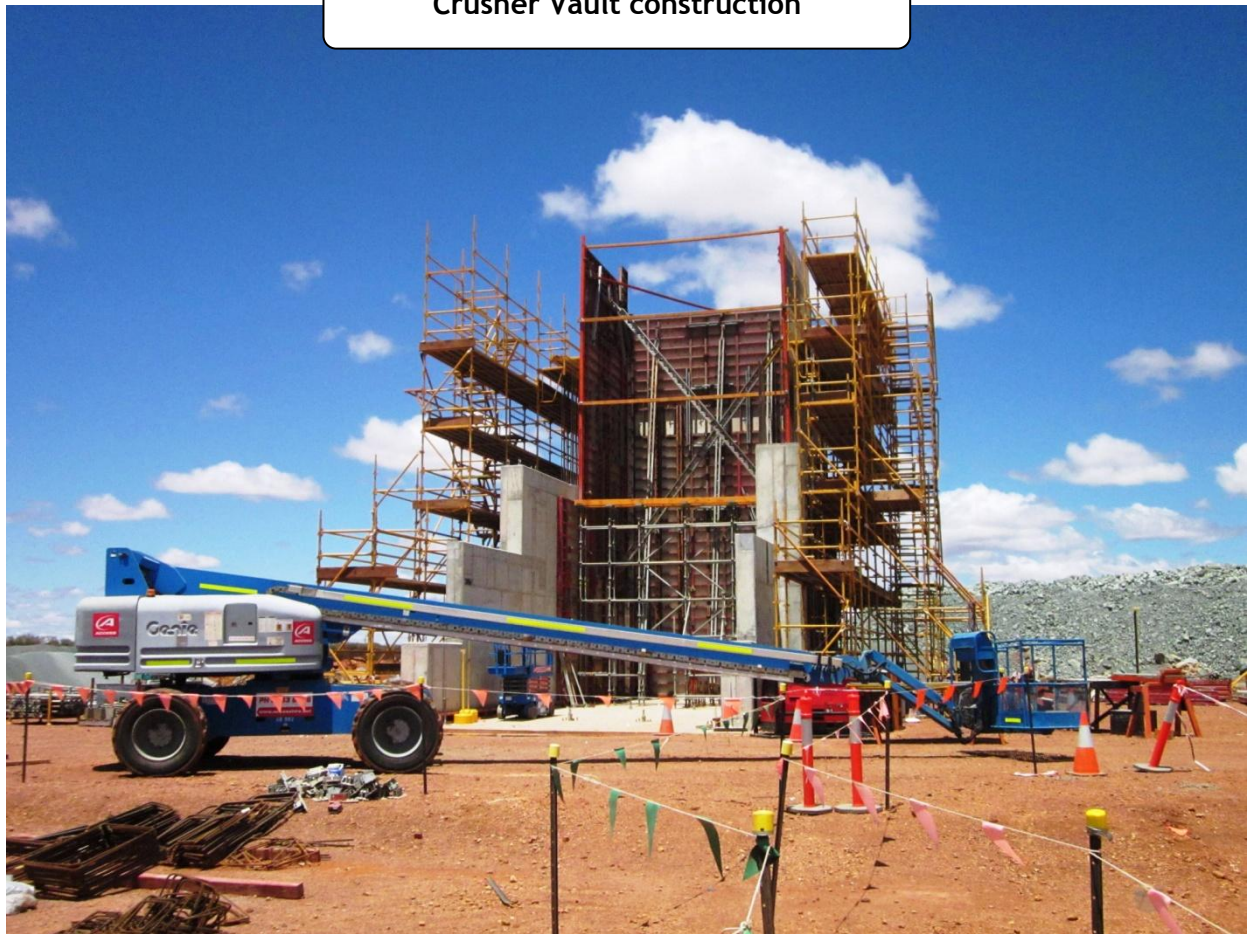
Crusher Vault construction
