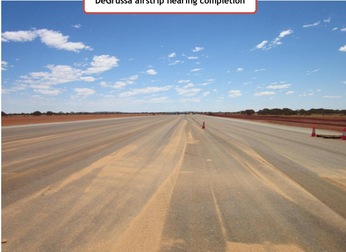
DeGrussa airstrip nearing completion
