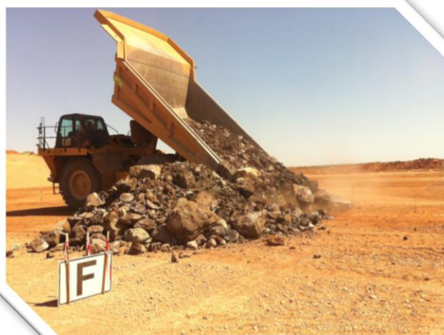
5.5 million bank cubic metres (bcm) of material mined to date Open pit 55 m below surface
