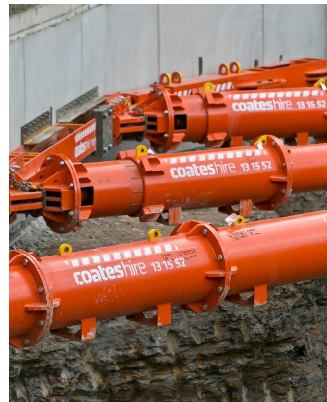
Coates Hire | Hydraulic Shoring | Sydney
