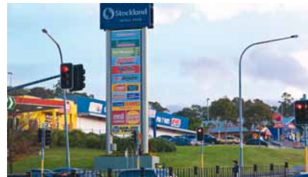
Shellharbour Retail Park
