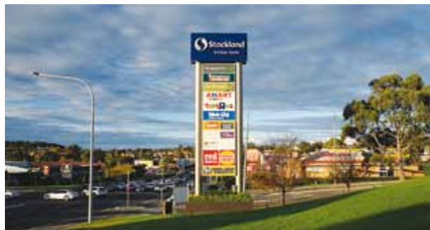
Shellharbour Retail Park
