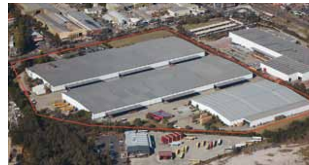
Forrester Distribution Centre
