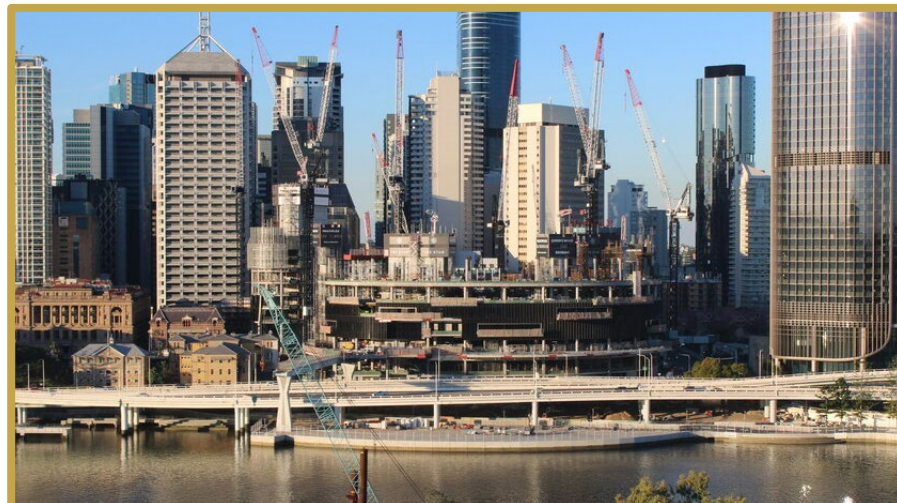
VIEW FROM SOUTH BANK – AUGUST 2021
